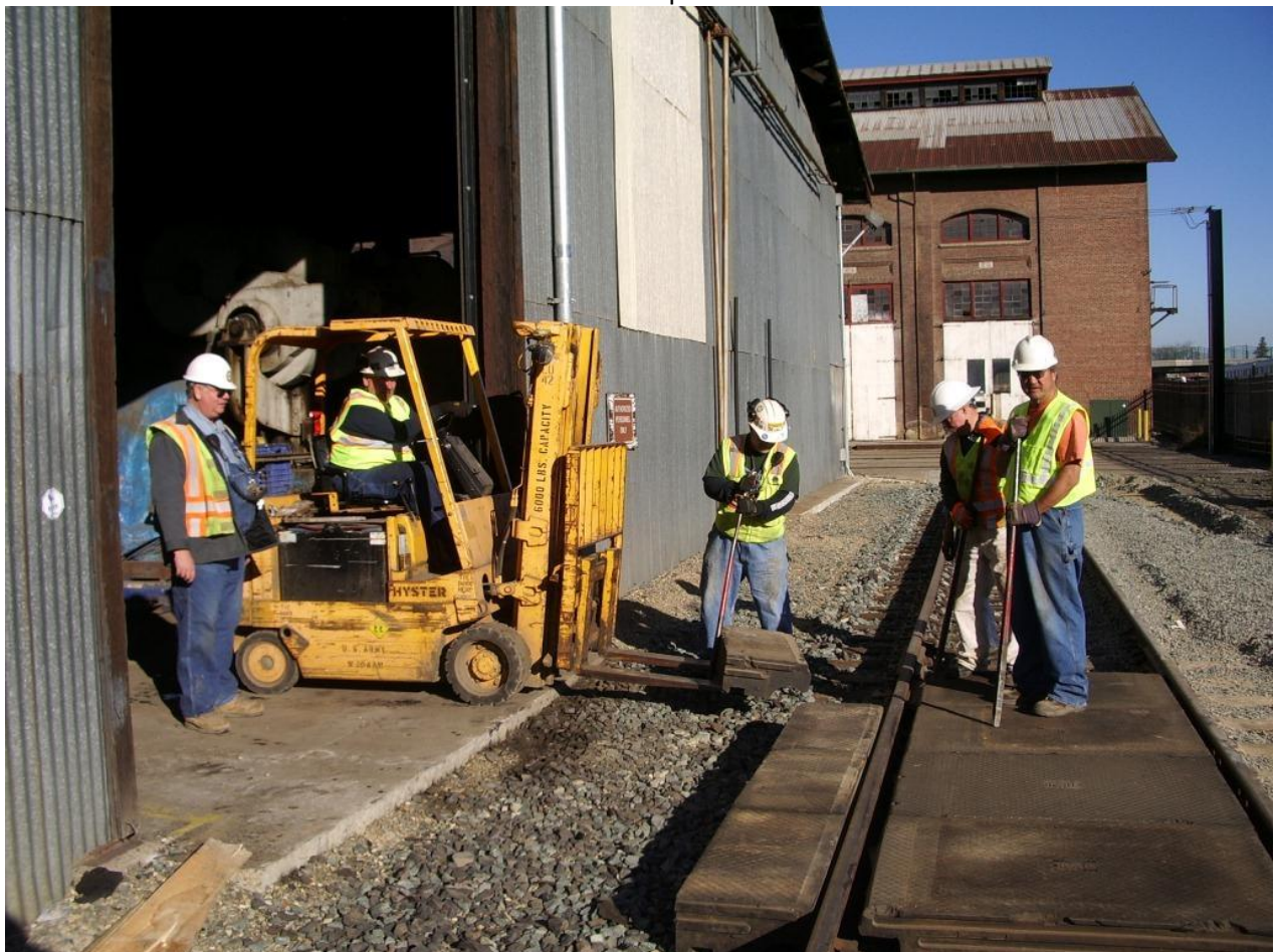
Chris, Harry, Mike F., Mike T., and John began laying the panels.
