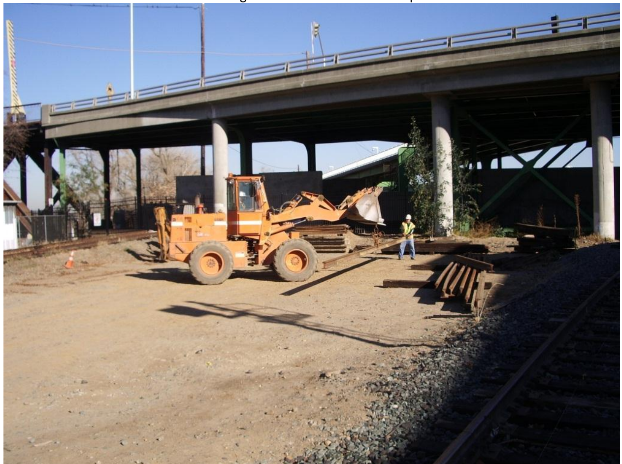
Mike F. guides a stick of rail being moved by Mike T. in the loader.
